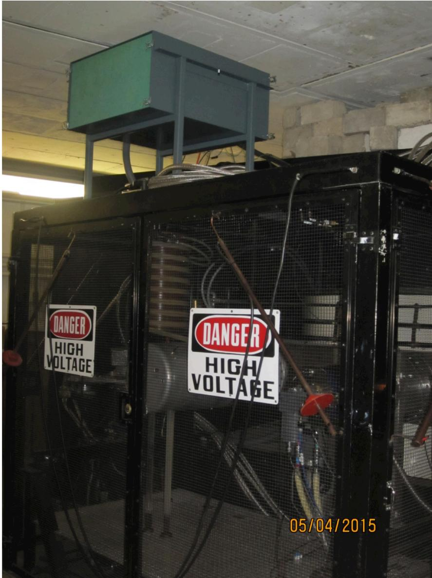
**FIG. 1.** The deflector power supply was relocated closer to the deflector above of the deflector cage. The supply is shielded from neutrons inside a box with 3 layers of 1" borated polyethylene panels.
